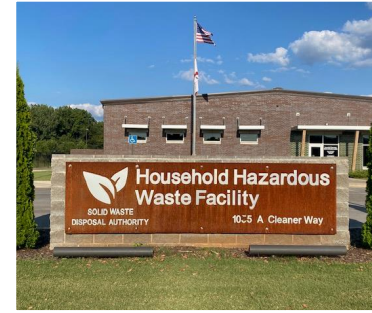
Household Hazardous Waste Drop-Off Facility
