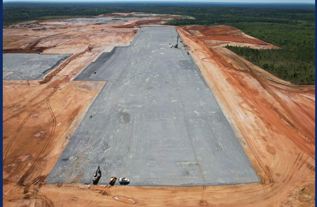
East view of site
